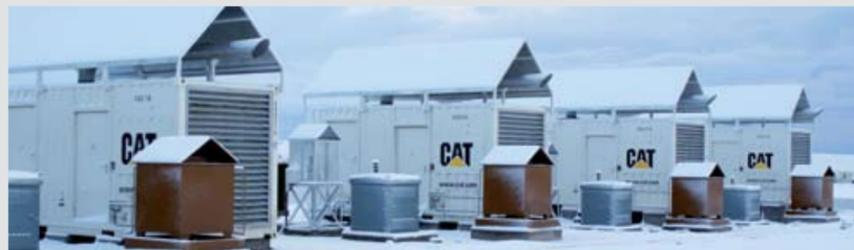
These 1 000 kVA Cat containerised gensets will supply prime power to run Plant 1 when a LEC shutdown occurs.
