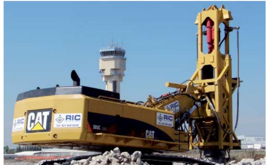
*RIC Africa's Cat 385C establishing the stone columns for the construction of OR Tambo International's new Airbus A380 apron.*
